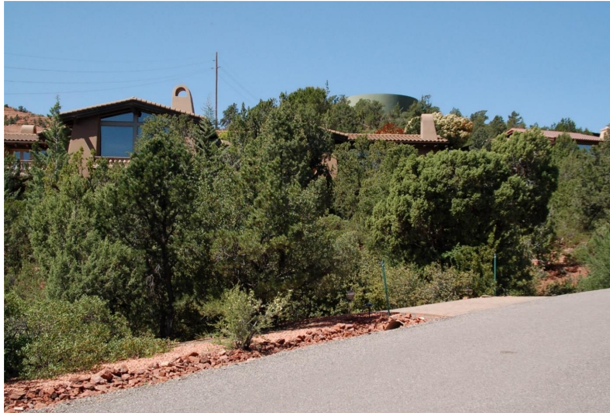
Shadow Rock Storage Tank, 700,000 gallons and visible from many of homes in the area.
