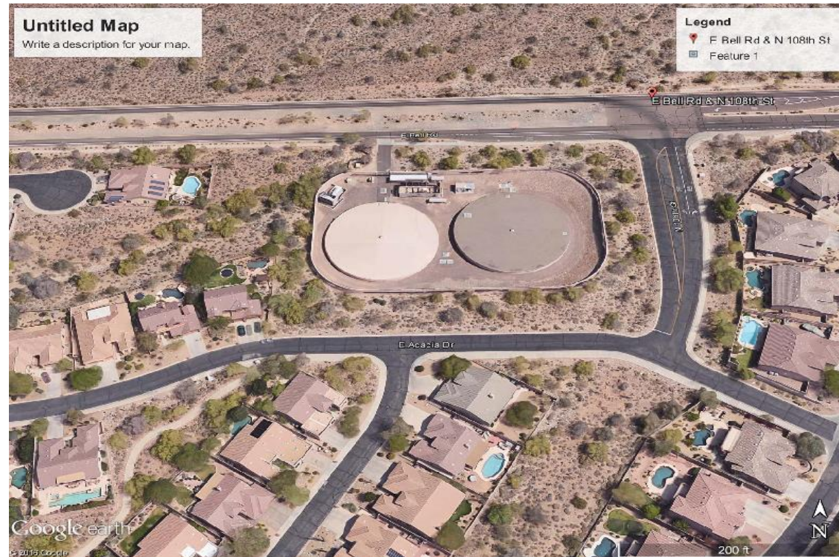
Scottsdale, Arizona Bell Rd. and 108 th St.
