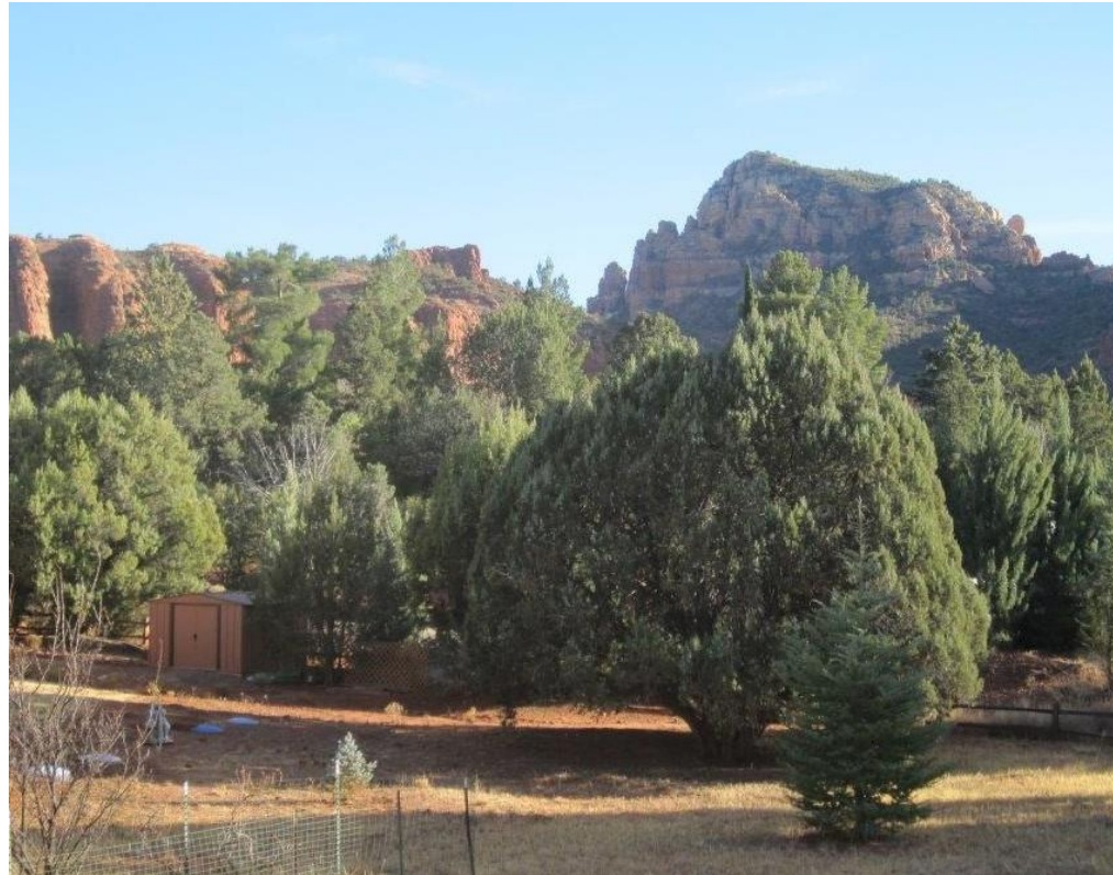
Broken Arrow Well No. 10 and arsenic removal facility. Located next to homes. Homes on two sides, located on State Route 179.
