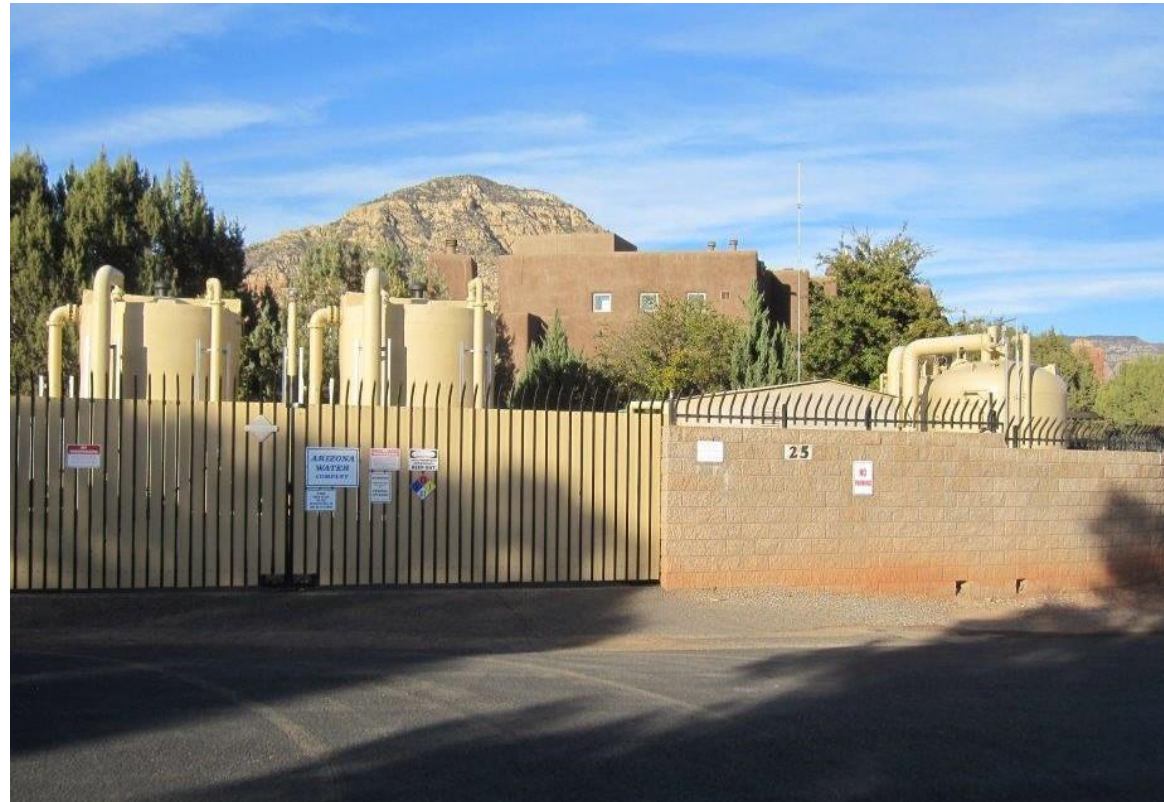
Southwest Center Well No. 8 and arsenic treatment plant a few feet from Adobe Grand Villas and down the street from City Hall.
